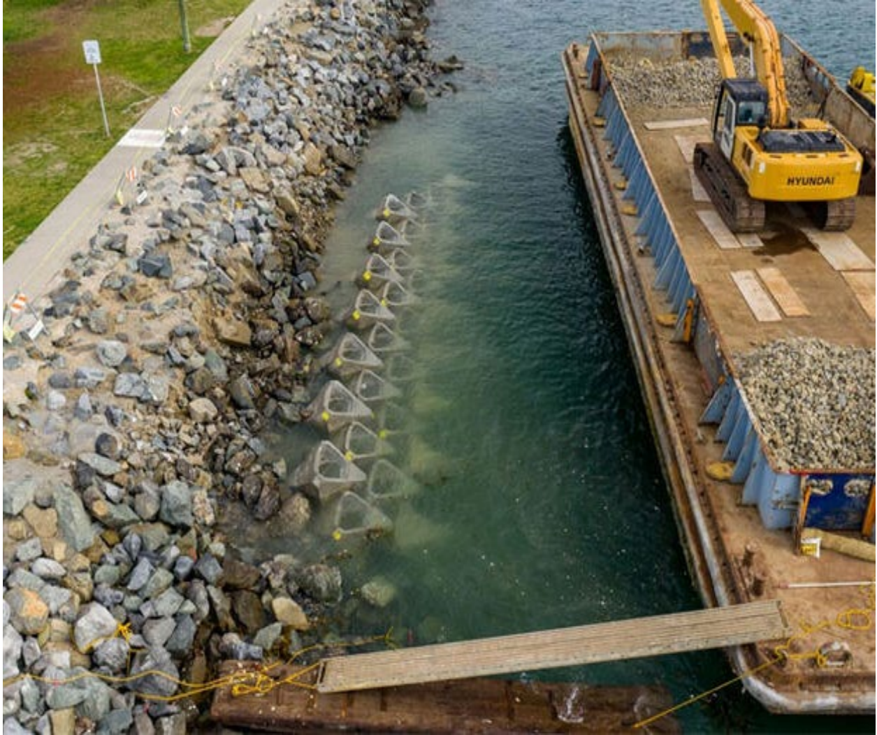
Figure I-22: Ecological armoring example: Eco-concrete Coast lock Blue Economy Pilot Project San Diego
